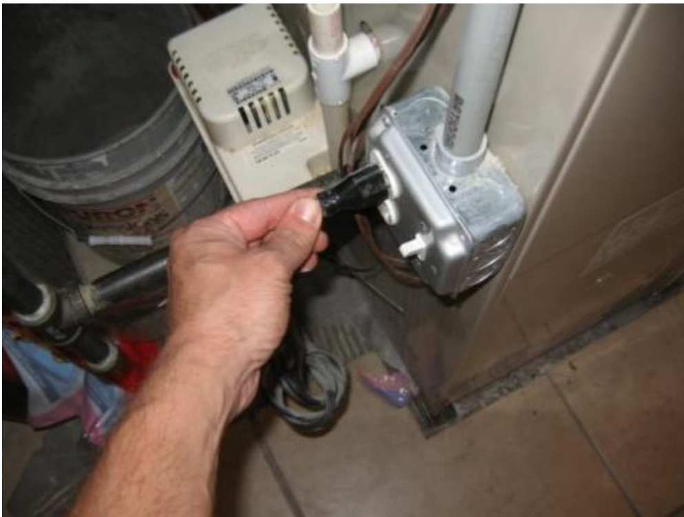
The condensate pump is plugged into an electric receptacle installed on the side of the furnace, next to the service shut-off switch.
