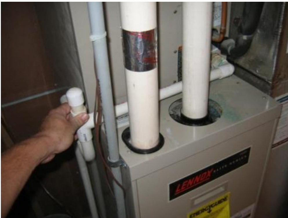
The home inspector is grasping the condensate drain pipe coming from the evaporator coil.
