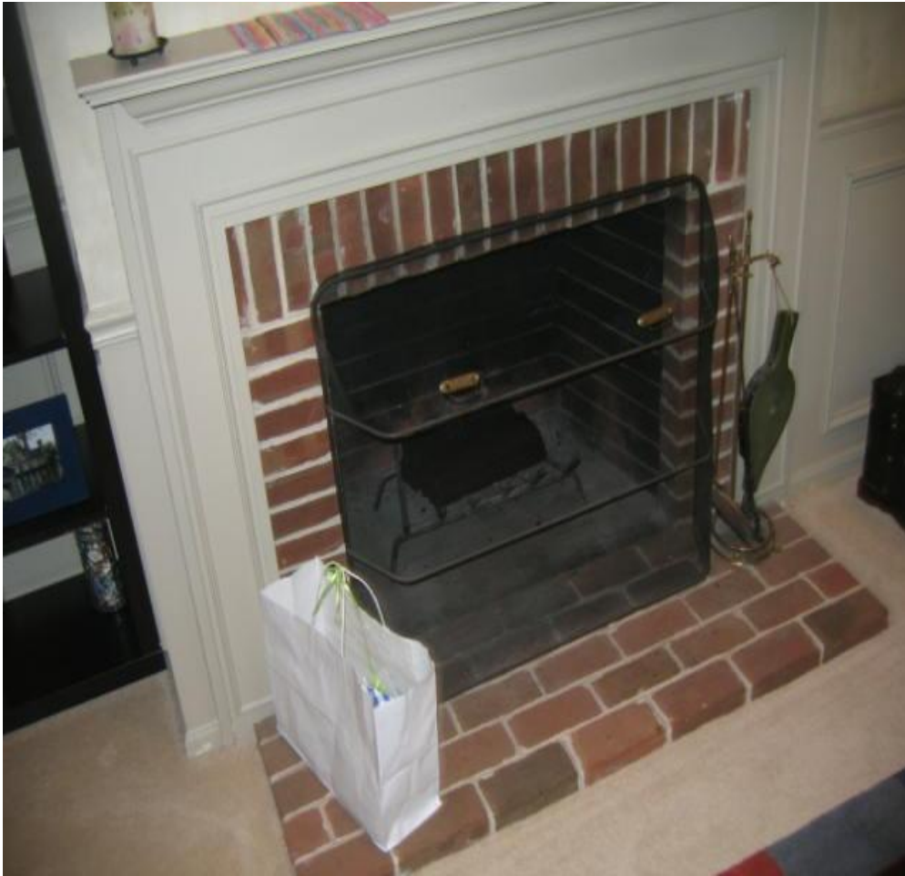
The inspection image above is of a masonry wood-burning fireplace in a house.
