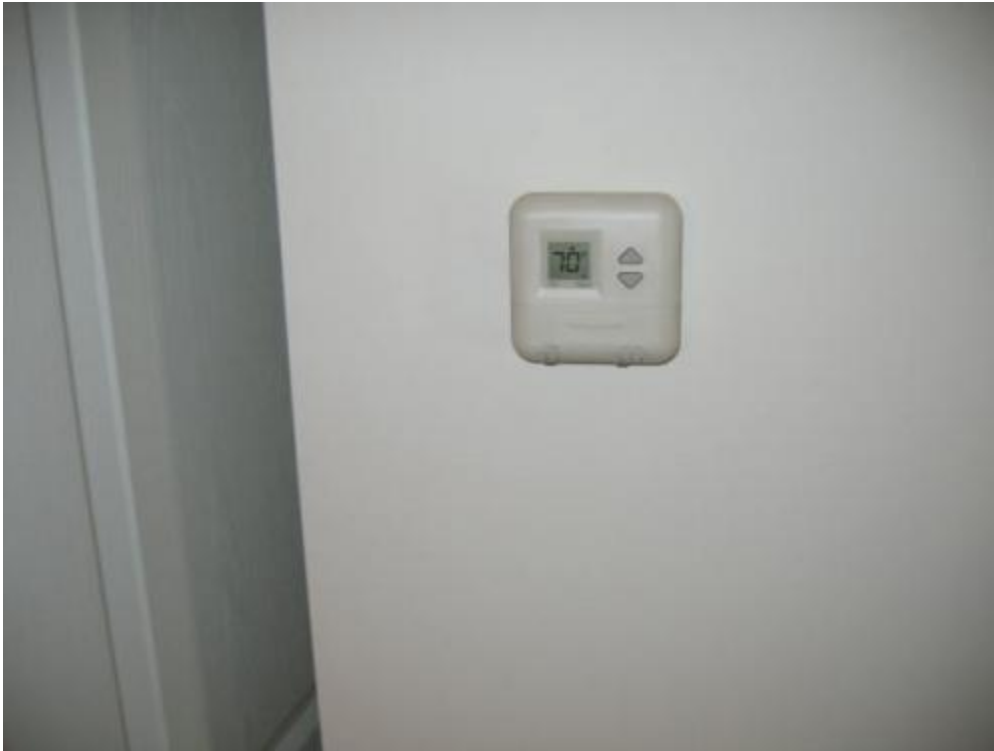
This is an inspection image of a thermostat, a normal operating control.
